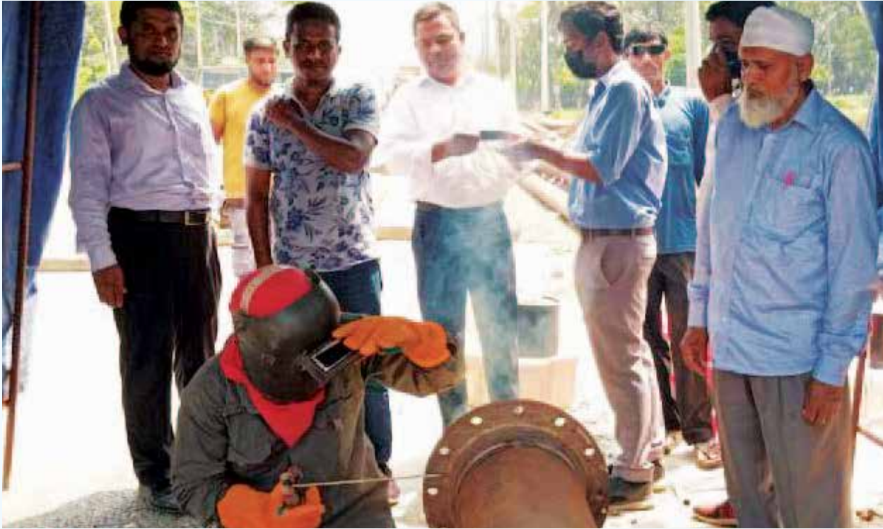
Welding activities going on for Construction of 4 bar & 10 bar gas distribution pipe line due to expansion of Cumilla - Noakhali highway.
